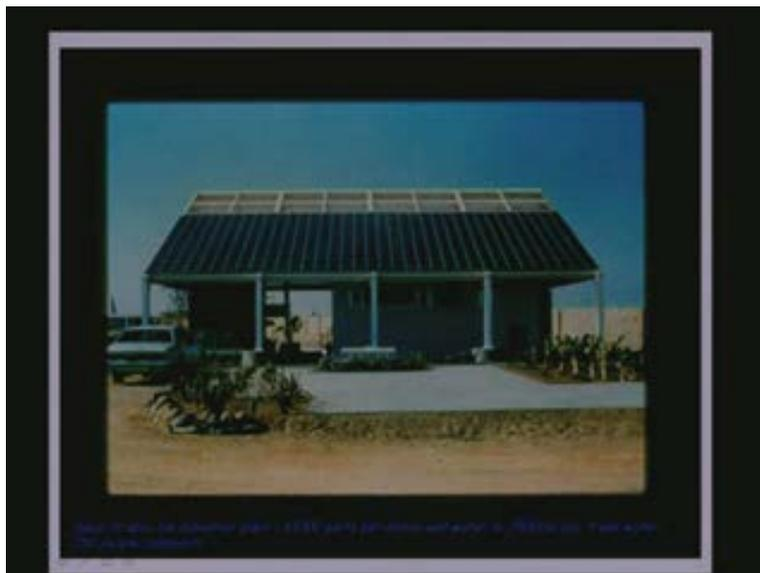
Here is another application where solar photovoltaic cells are found used. This is in the middle-east. This building is a desalination plant which takes in the sea water, sea water contains lot of salt and it is desalinated by reverse osmosis process.
