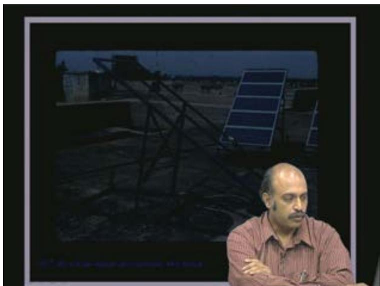
These are also some other photovoltaic modules. These are polycrystalline modules. These are 44 watt modules and of course (Refer Slide Time: 15:25) these are mounted on top of our laboratory here to do experimentation.
