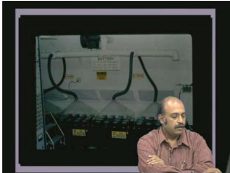
The photovoltaic array charges up this battery bank and from this battery bank it goes through a converter to supply the various loads **as I showed** or as I have told earlier in the block diagram.
