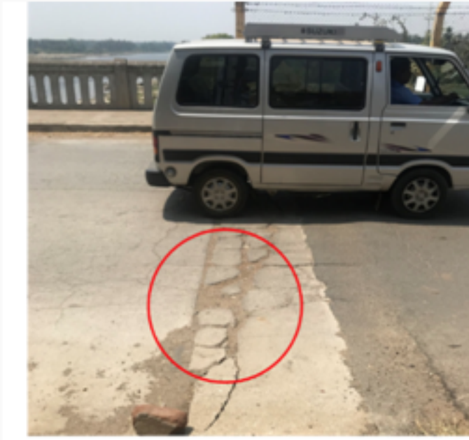
Bridge Joint Approach road
