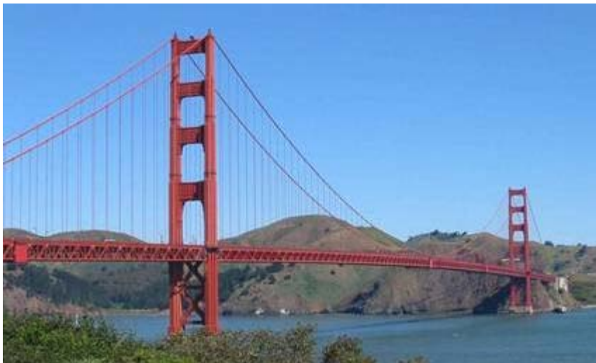
Figure 3.2 A suspension-cable bridge (Golden gate bridge, San Francisco , USA)
