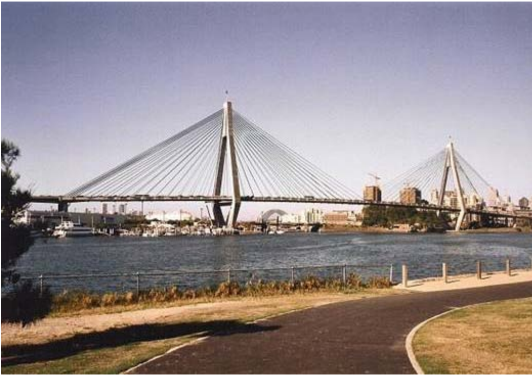
Figure 3.3 A cable-stayed bridge (ANZAC bridge, Sydney , Australia )
